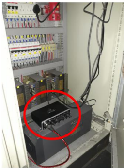
Fig. 5. Behringer Uphoria UMC202HD in TBR Drum test machine.
